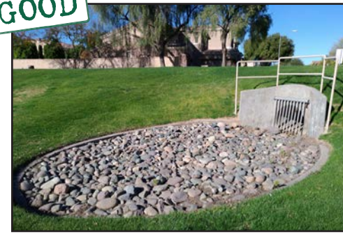
Storm Water Basins & Headwalls
