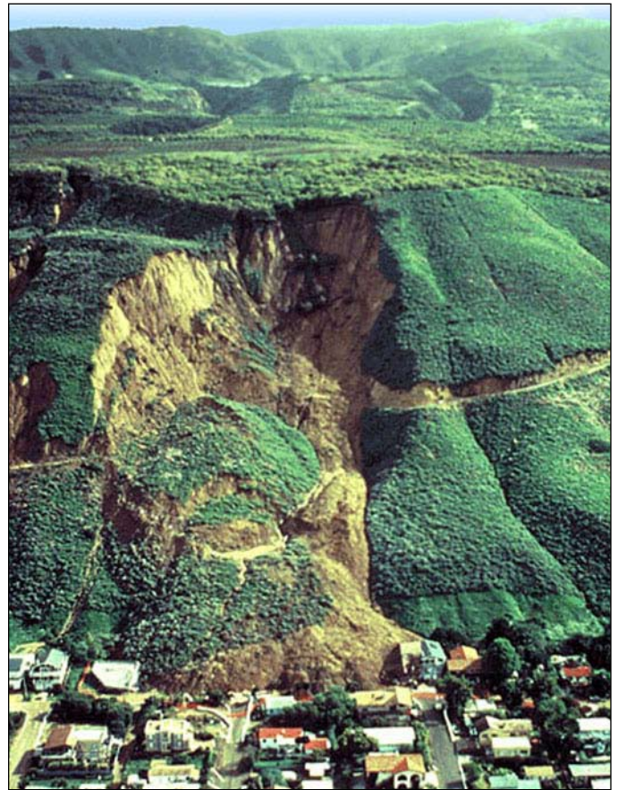
In La Conchita, CA, landslide and debris flow occurred in the spring of 1995. Many people were evacuated because of the slide and the houses nearest the slide were completely destroyed. Fortunately, no one was killed or injured. (Photo by R.L. Schuster, U.S. Geological Survey. landslides.usgs.gov )
